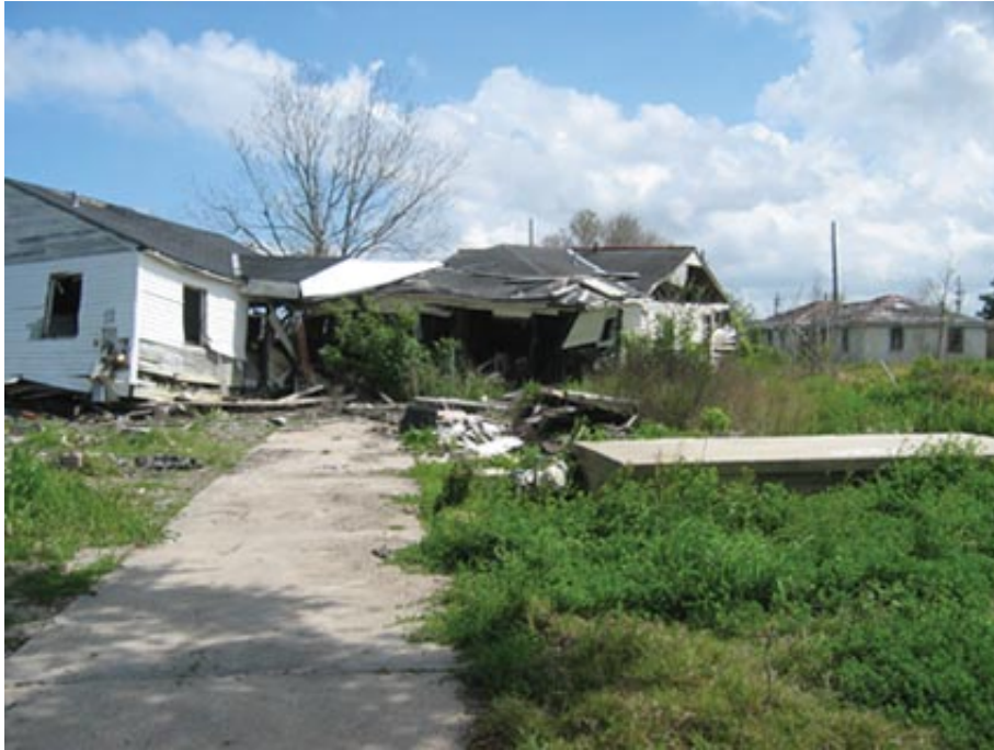
Figure 10.14 Destroyed House in the Lower Ninth Ward, New Orleans.
